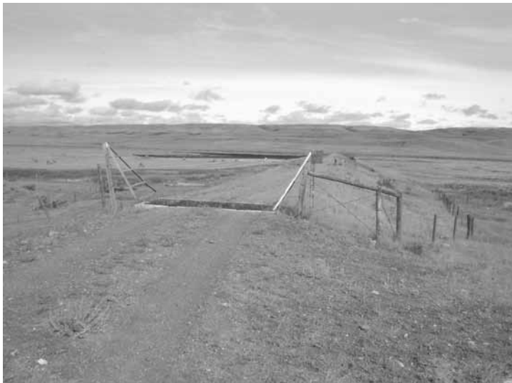
Dam at the west end of Cypress Lake, southwest Saskatchewan. The road runs along the top of the dam. Cypress Lake is a reservoir serving several irrigation districts in southwest Saskatchewan.
