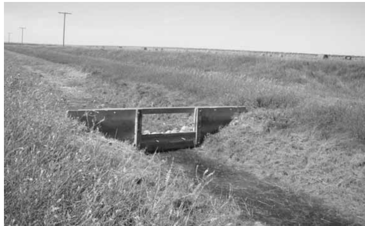
Water flow control gate at Miry Creek Irrigation District, near Cabri, Sask.
